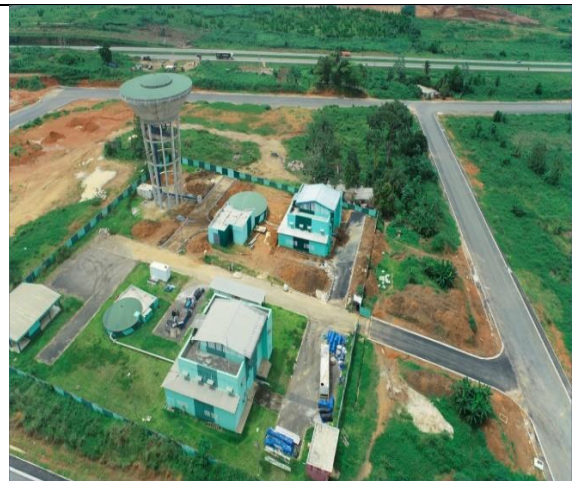
Image showing a water tower and a neutralisation and disinfection station at PK 24 Akoupé-Zeudji
