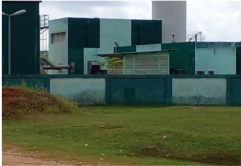
Figure 5-59 SODECI Treatment plant in Adonkoi I, 2022
