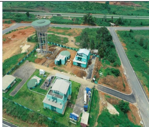
Image showing a water tower and a neutralisation and disinfection station at PK 24 Akoupé-Zeudji
